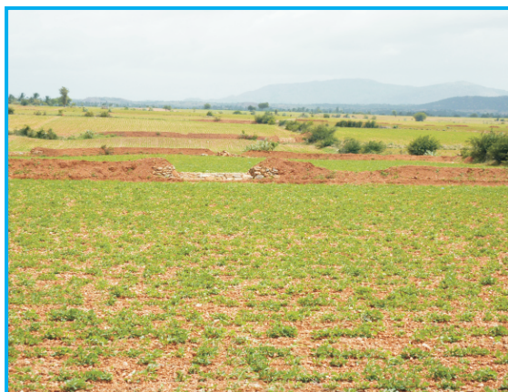
Plate 10: Series of field bunds with waste weirs established in arable land. Sketch of loose stone revetment alongside.
