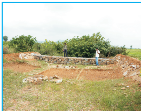
Plate 7: Views of gabions made in the lower reaches to reduce velocity of flowing water
