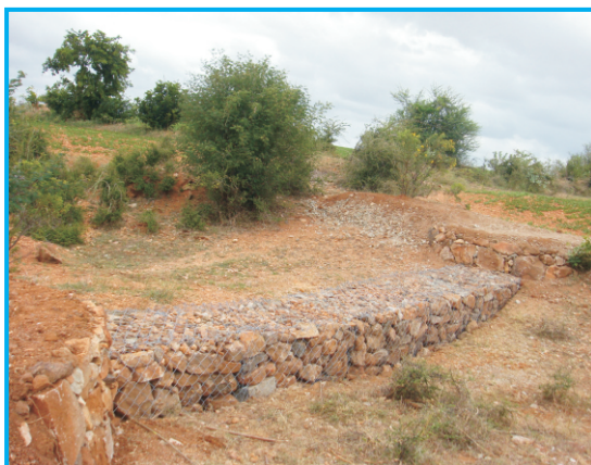
Plate 7: Views of gabions made in the lower reaches to reduce velocity of flowing water
