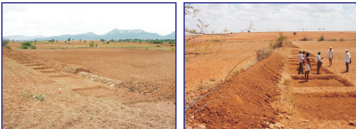
Plate 11: View of construction of bunds using soil from borrow pits
