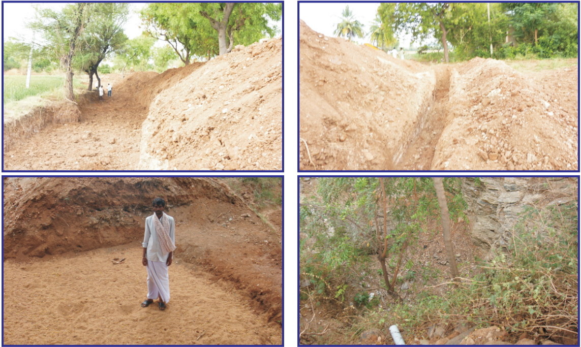
Plate 24: Views of the channel leading to a recharge filter pit and open well in which surplus water is safely diverted.
